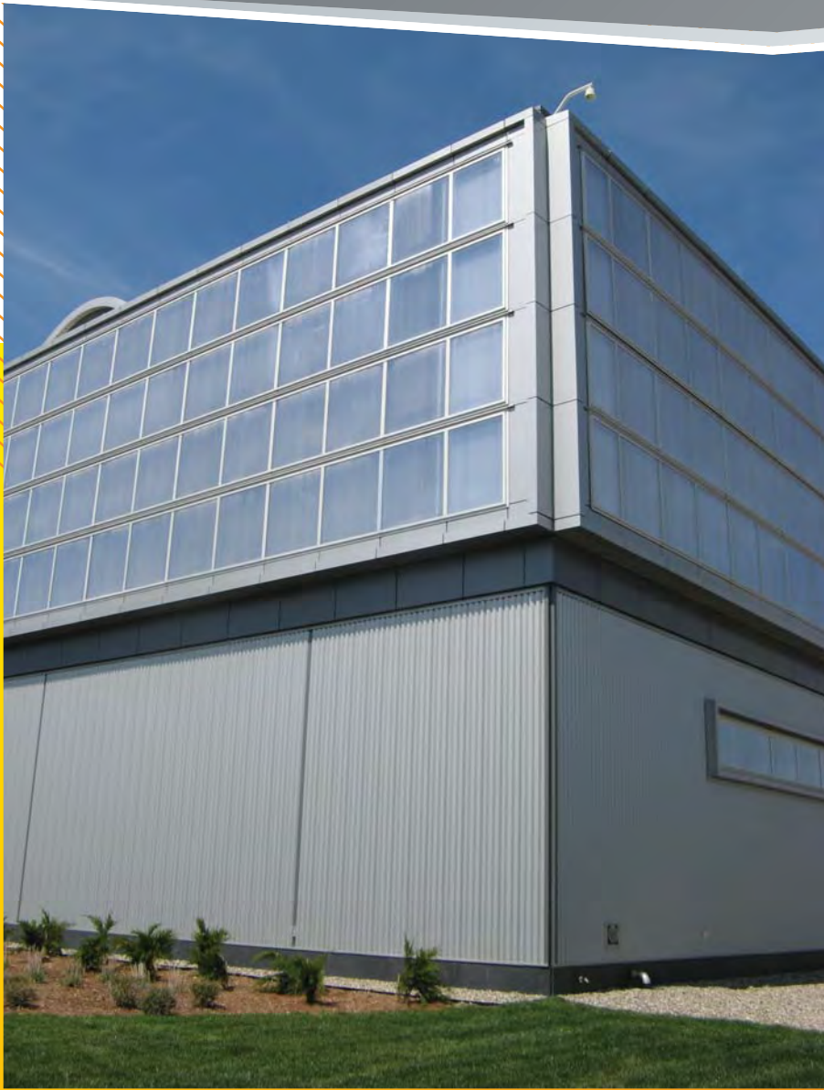
PROJECT: Net App Center ARCHITECT : O'Brien Atkins
