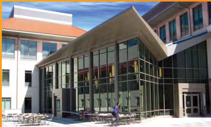
PROJECT: Emory Candler School of Theology ARCHITECT : Collins, Cooper, Carusi Architects
