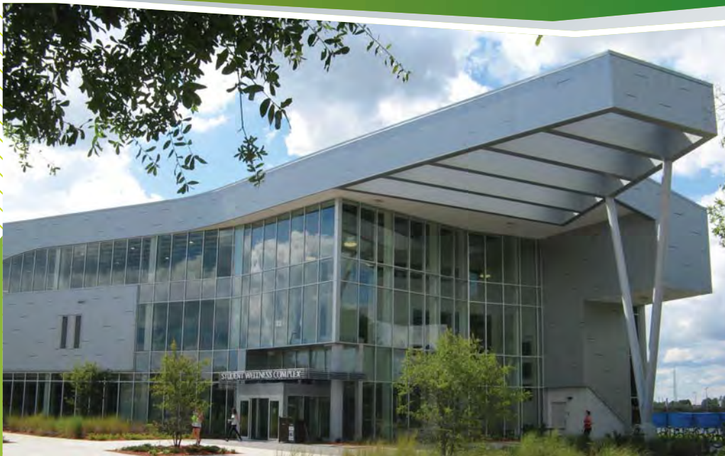
PROJECT: Univ. of North Florida ARCHITECT : PSA-Dewberry Architects
